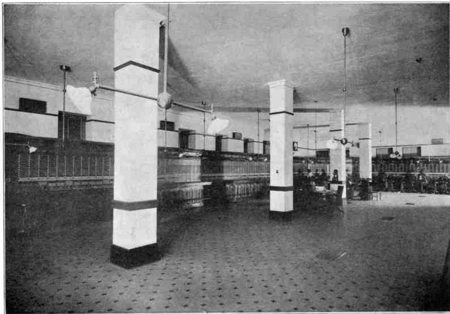
Fig. 424. Subscribers' Board. Chelsea Office, New York City View full size illustration.
