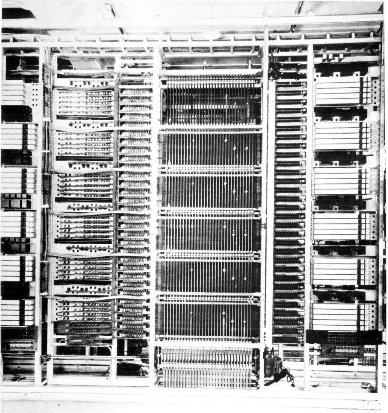
Figure 5-1 Typical Panel Dial Selector Frame
