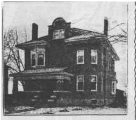
RESIDENCE OF W. S. WISNER Built by Secord & Sons.
