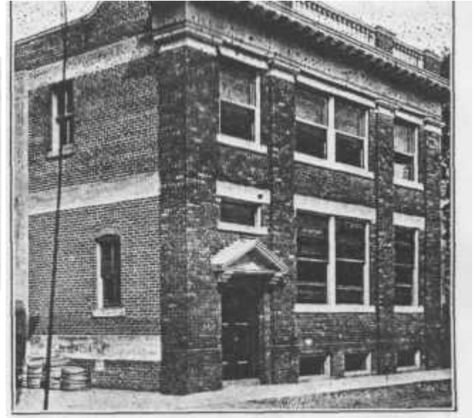
Canadian Machine Telephone Company's Exchange and Office, Brantford
