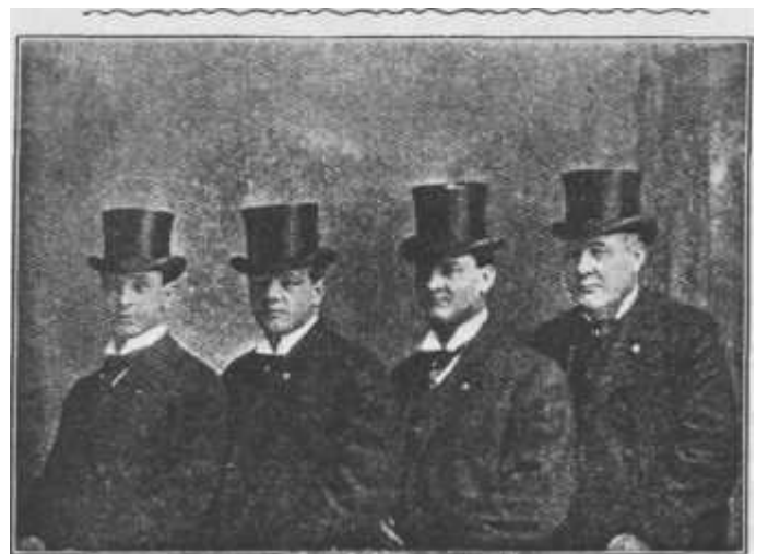
HARRY JOHNSON FRANK C. JOHNSON, Jr. WALTER JOHNSON FRANK C. JOHNSON, Sr.
